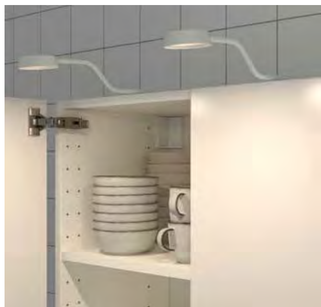
Over cabinet lighting
